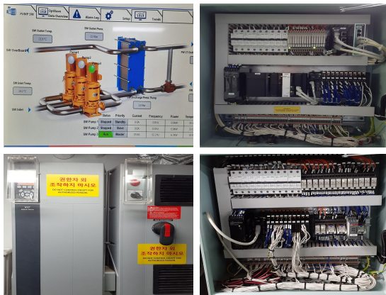
[Fig. 4] Control Panel and Mimic System of ESS.
