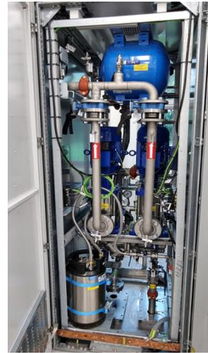
[Fig. 5] Cooling unit of AC drive.
