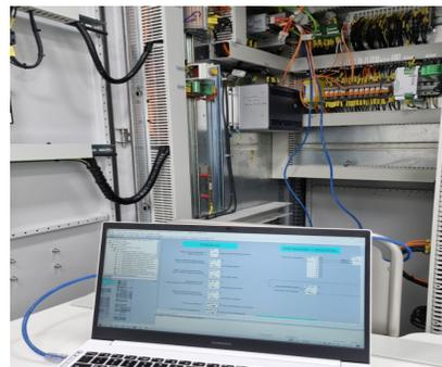
[Fig. 6] Communication between computer and AC drive.
