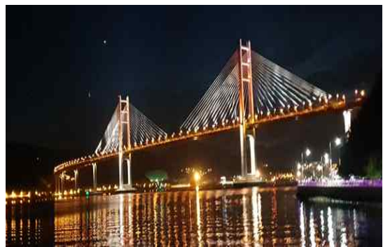
[Fig. 5] Case of confusion between Geoga Bridge and port lighting.
