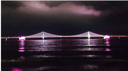
(a) Gwangan Bridge
