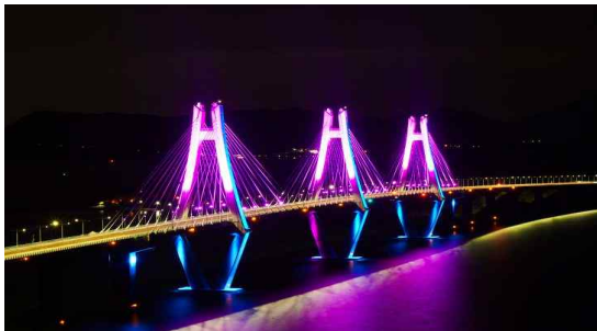
(b) Geoga Bridge
